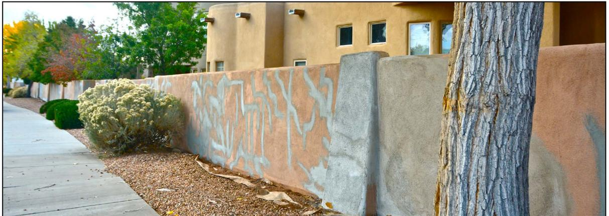
Current wall repair work began in early November on the masonry wall installed adjacent to Rio Grande Blvd. This work consists of repairing cracks in the masonry and resurfacing to provide a uniform color and textured surface. This project should be finished as this newsletter goes to press.
